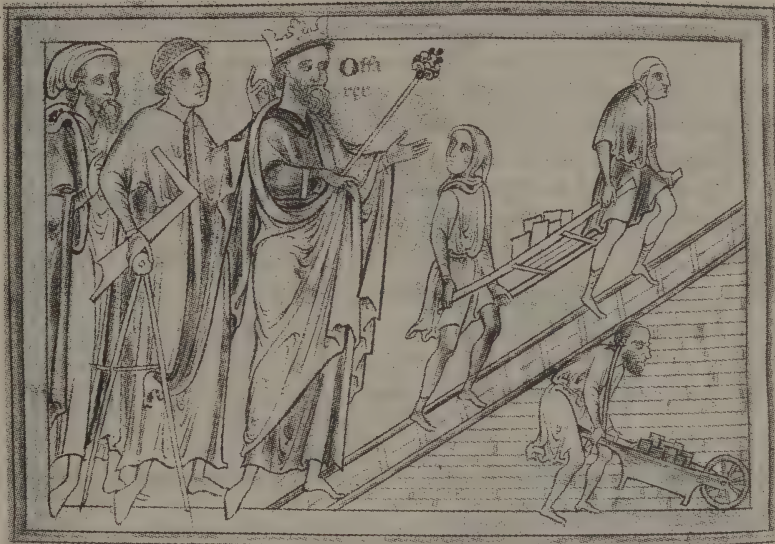
A construction scene, dating about 1250, showing both a stretcher and a wagon-type wheelbarrow being used. The strap across the porter's shoulders reduces the load on his arms.
